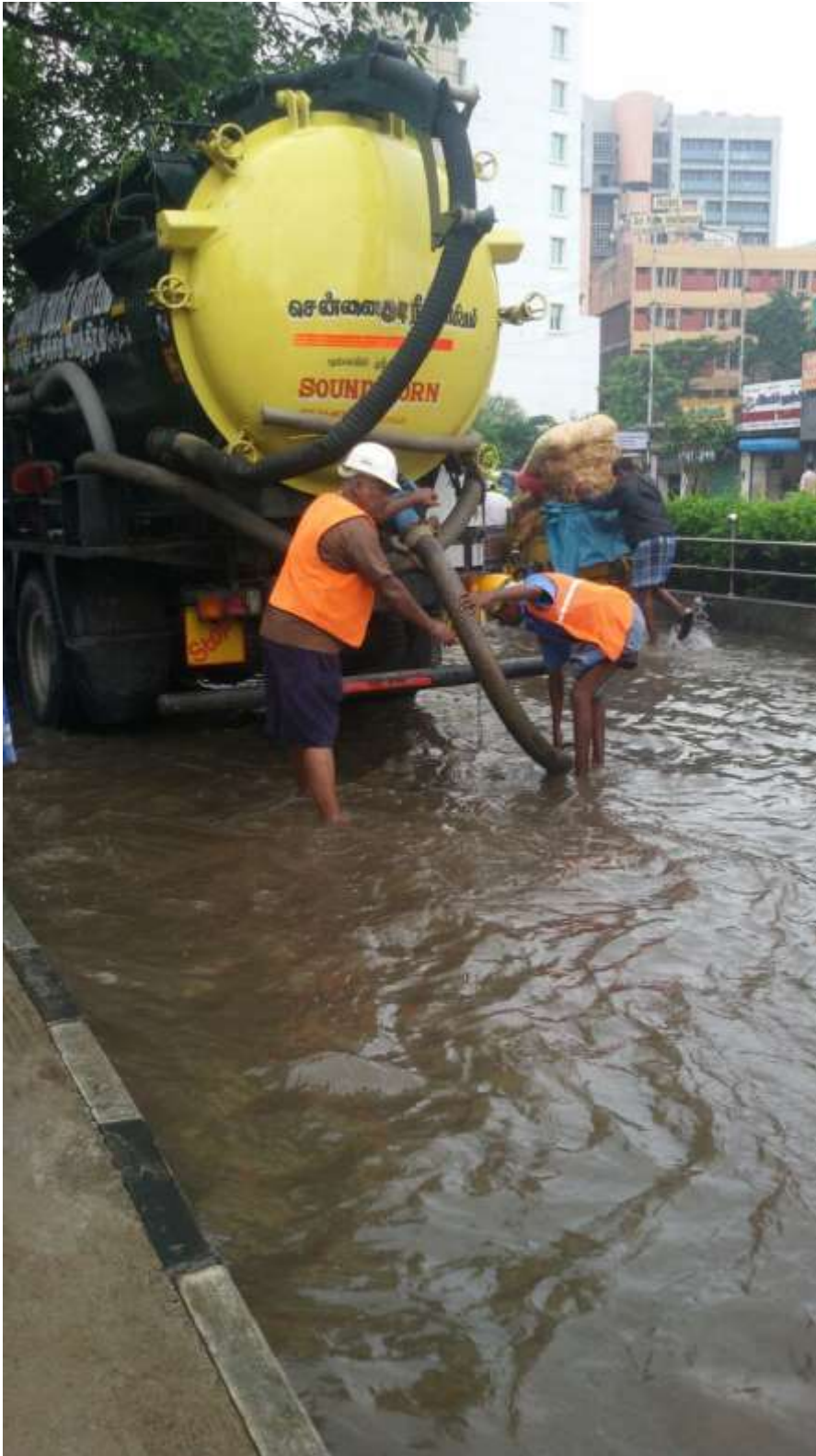
Dewatering stagnated rainwater using super sucker at Gandhi Irwin Road near Egmore Railway Station
