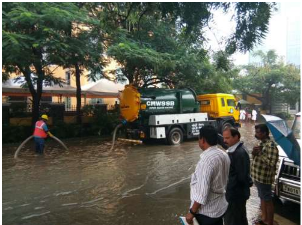
Dewatering the rain water at MRC Nagar
