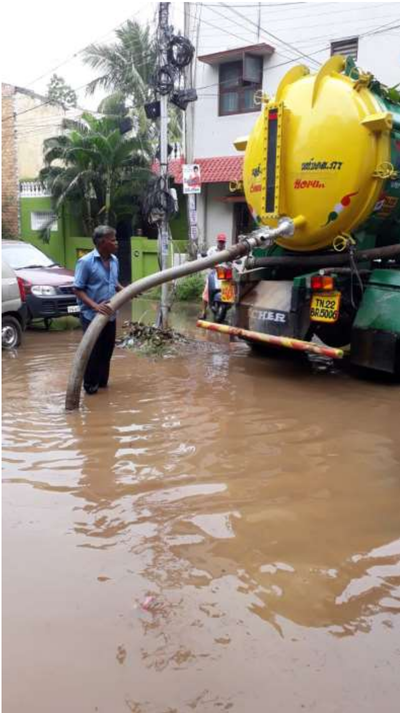
Pumping of stagnated rainwater using super sucker at TNHB 7 th street in Depot 177 Area XIII
