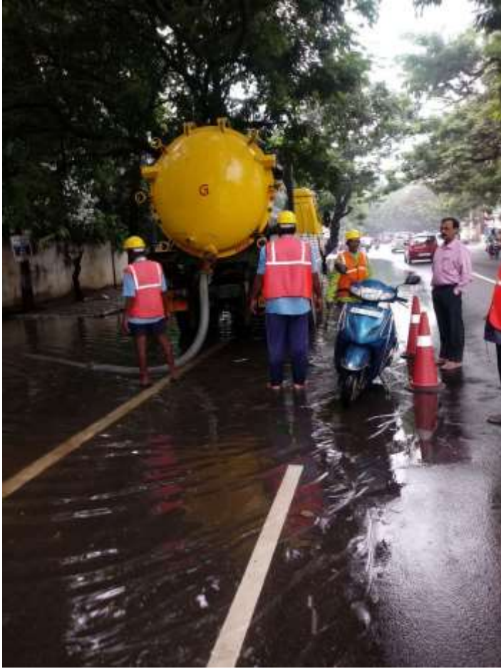
Area 8, Super sucker working at 1 st Avenue, Anna Nagar.
